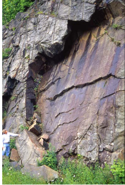
Figure 3. Site of rock fall along joint surface in July 2000.
